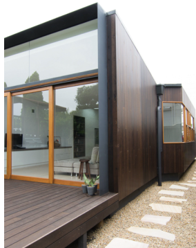
Flushed lining to the rear extension as the deck extends from the interior.
