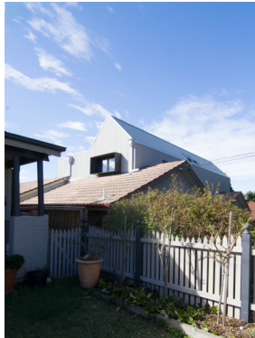
The second storey addition as seen from street view.
