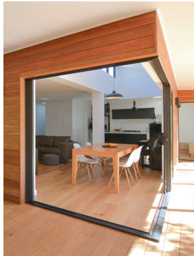
Pocket sliding doors to create a seamless extension of the dining space to the verandah.
